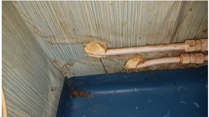
Pipe grommets in the wet area.
