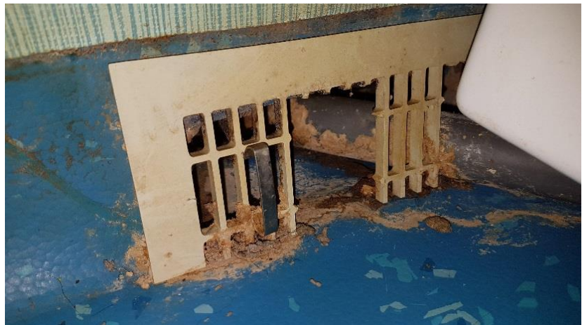
Wall drains since year of construction.
